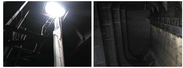
Fig. 3. (left) Oil tanker manhole entry point. (right) Typical oil tanker cargo hold.
