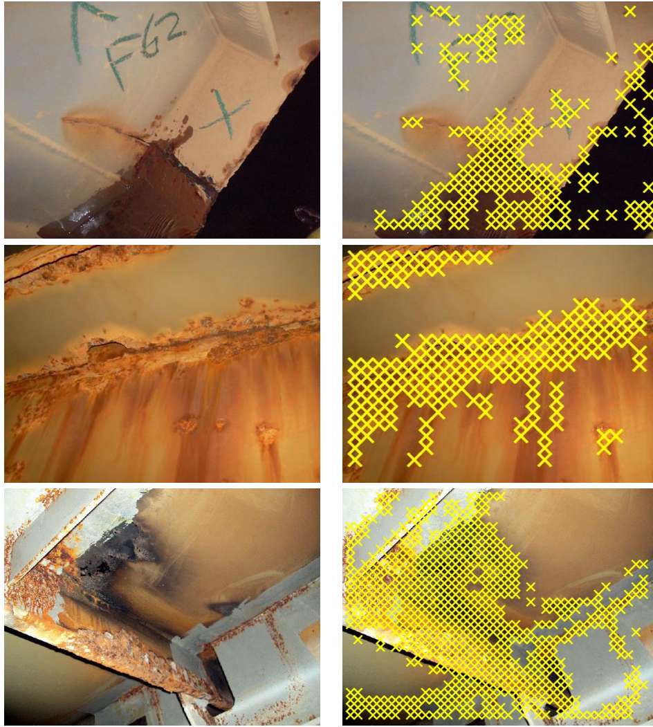
Fig. 1. Test images and patches labelled as coating breakdown
